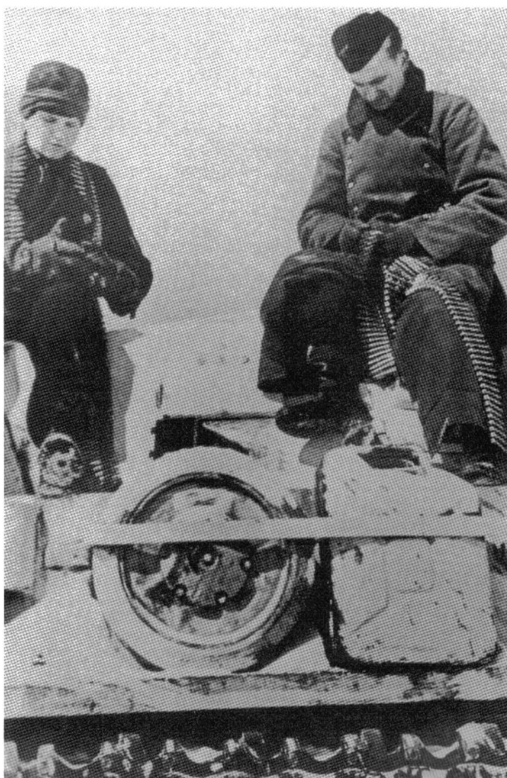
Two photos of a winter whitewashed Pz.Kpfw.IV Ausf.F1 being refueled and having its MG ammunition replenished during the winter of 1941-42. This enterprising crewman is utilizing a captured Soviet gas mask filter canister and hose as funnel to assist in the refueling process.
