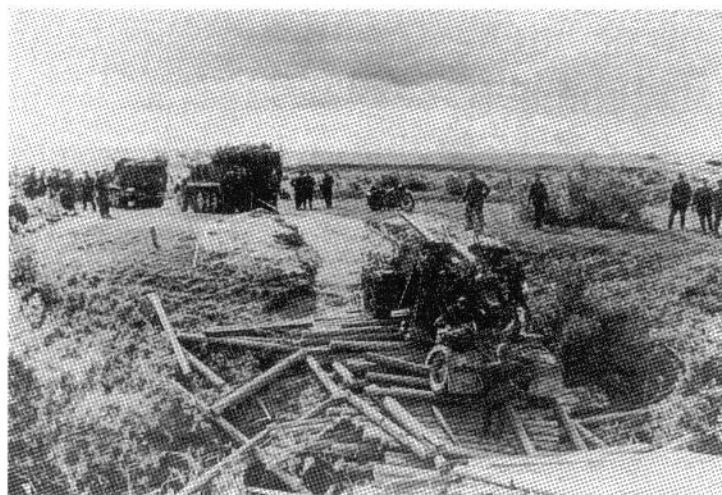
Two Sd.Kfz.8 half-track prime movers attempt to retrieve an 8.8cm FlaK18 anti-aircraft gun that was on a crude log bridge that has collapsed from the weight. The momentum of the German advance taxed the engineer units to their limit as the Army spread out over a much wider front with longer lines of communication and supply than in the previous year. The photo was taken near Stalingrad in August, 1942.
