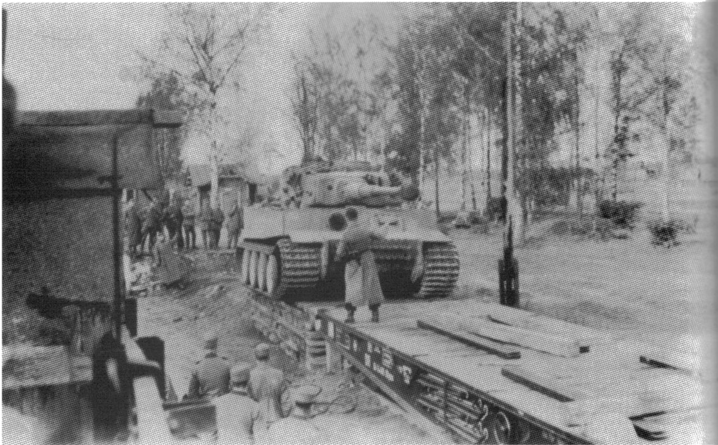
Two photographs of one of the first nine Tigers of s.Pz.Abt.502 being unloaded from a railroad flatcar at its destination in Russia in the late autumn of 1942. It was produced in early November 1942 as it is fitted with the new standard track but still has not been fitted with the side track guards. Not visible in the photos is the Pz.Kpfw.III stowage bin carried on the rear of the turret. The tactical number '102' has been painted in white outline on the side of the turret along with a large white outline Balkenkreuz on the side of the hull just ahead of the last outside roadwheel and the emblem of s.Pz.Abt.502, a white outline 'Mammut', on the front plate. Though it appears a light color, it is still in its original dark gray paint with a heavy coating of dust.
