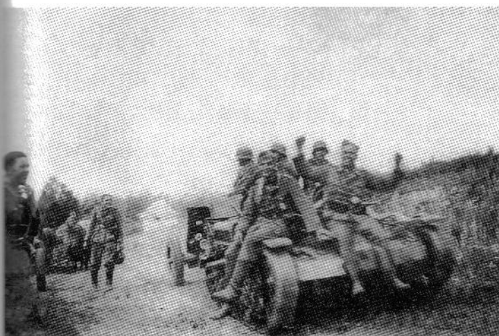
Another 3.7cm PaK35/36 gun crew enjoy a ride on a Renault UE 630(f) being utilized as a gun tractor. This little vehicle was perfect for short distance moves but would have been extremely uncomfortable on a long march.
