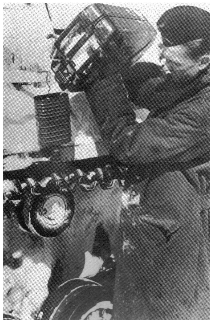
Two photos of a winter whitewashed Pz.Kpfw.IV Ausf.F1 being refueled and having its MG ammunition replenished during the winter of 1941-42. This enterprising crewman is utilizing a captured Soviet gas mask filter canister and hose as funnel to assist in the refueling process.
