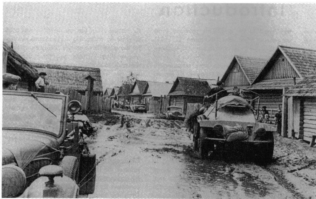
Vehicles of a divisional reconnaissance troop struggle down a muddy road through a Russian village in July, 1941. The armored car on the right is an early version of the kleine Panzerfunkwagen (Sd.Kfz.261). This one is a standard Sd.Kfz.221 that has been fitted with a frame antenna and additional radio equipment and still carries the standard MG34 armament. Later versions were built on the chassis of the Sd.Kfz.223 and were unarmed. Markings on the left mudguard indicate it belongs to 8.Panzer-Division. The vehicle on the left is a BMW 326 two-door convertible, one of many types of civilian cars utilized by the Wehrmacht.
